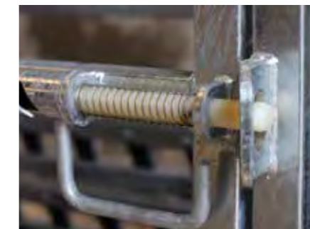
7. NEW NYLON ROTARY BOLT For noise reduction
