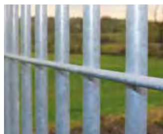
WELDED CROSS BAR FOR STRENGTH
