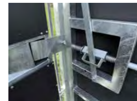
9. SLIDE OVER PLATES Seamless transition between race sections
